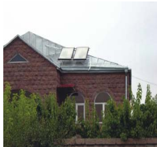
Figure 12. Solar Water Heating System, private house
