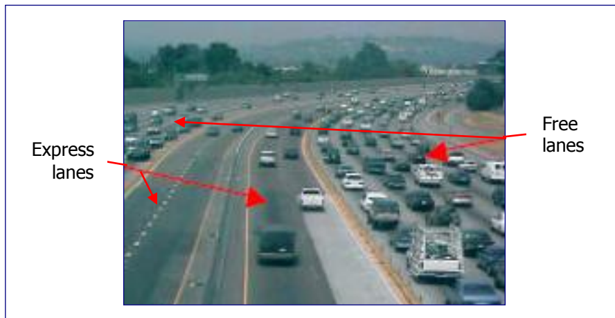
Figure 18. Express and general purpose lanes of SR 91
